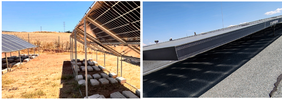
Fig. 1. Mounting conditions of bifacial PV modules/systems. The amount of shading depends largely on the module's ground clearance.
