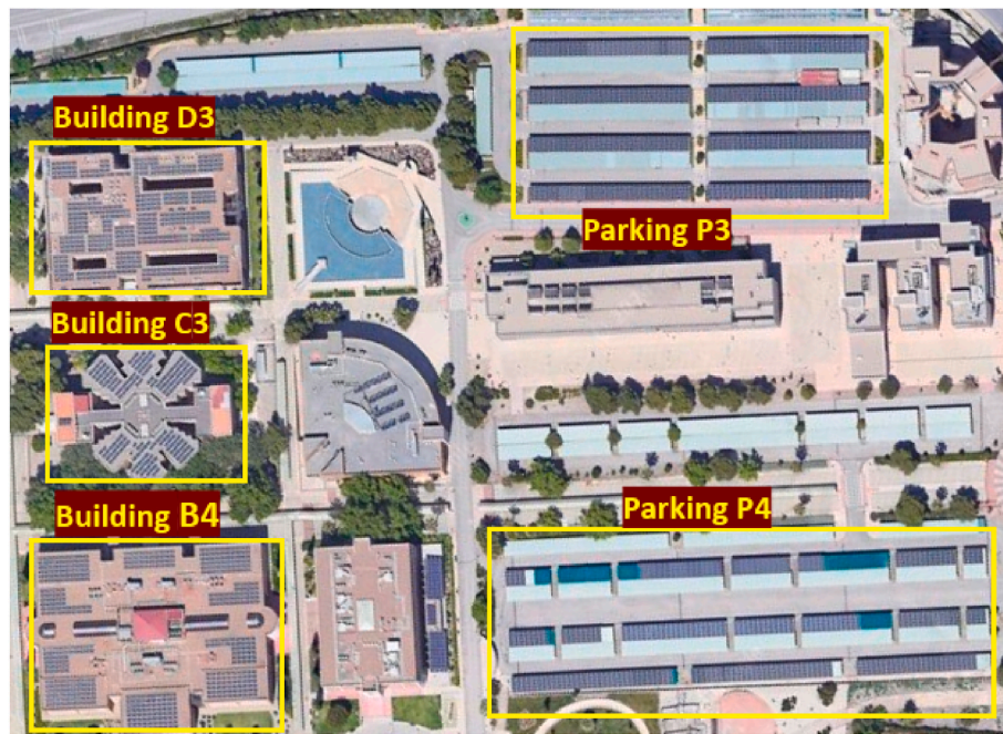
Fig. 1. Rooftop PV system installed at University of Jaén which is composed of five Rooftops PV or subsystems installed on the Rooftops of buildings B4, C3, D3 and parking lots P4 and P3.
