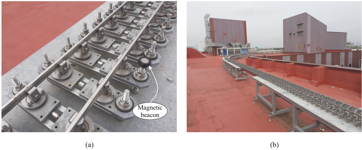
Figure 1: (a) Track sleepers. (b) Track overall view
