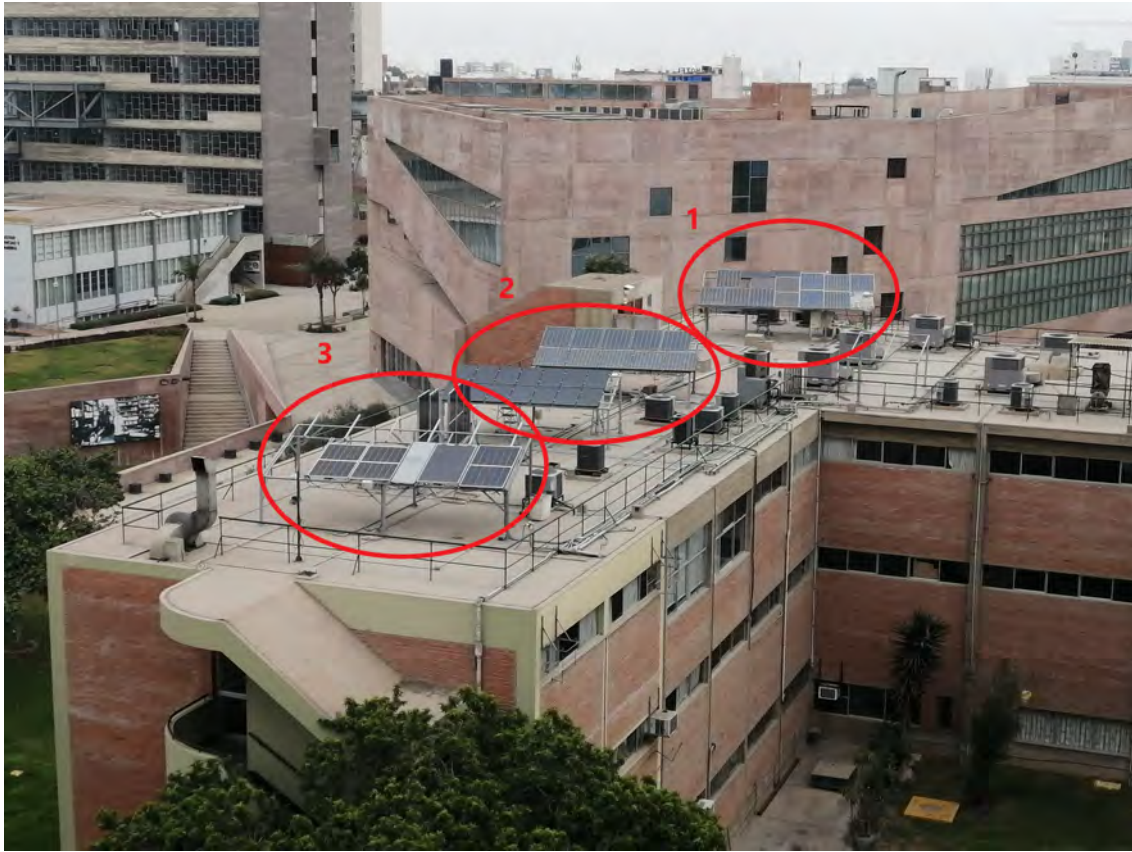
Figure 5.1: PV Research Laboratory at PUCP.
