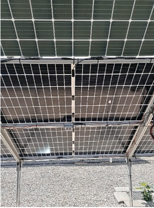
Fig. 2. Back view of the bifacial PV modules, reference cell and pt 100, [23].
