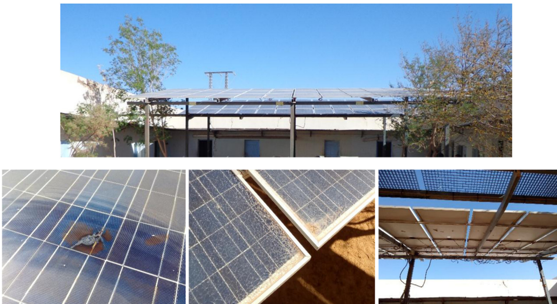
Fig. 6. Regional hospitals and School of Nursing PV installations showing similar problems regarding operation and maintenance: a) El Aiun, overall view of the installation and detail of some issues, such as sand within the connection boxes and shading by misalignment of the PV structures; b) Awserd, problems with the PV generator showing burnt cells in the modules and poor wiring; c) Smara, burnt cells and broken glasses in the PV modules, poor wiring; d) Dakhla, overall view with a fixed antenna in the middle that provides shading over the PV modules, poor wiring and not appropriate location for the batteries; and e) School of Nursing, showing different types of PV modules with burnt cells, poor wiring.
