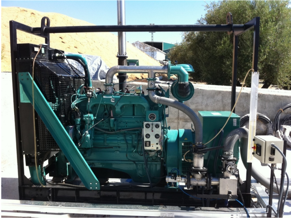
Figura 6.3. Picture of the engine model Cummins G-855-G (Úbeda).
