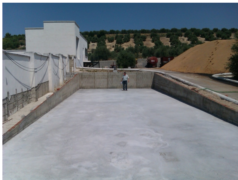
Figure 6.5. Shed required for GAS 70 Plant (Úbeda).
