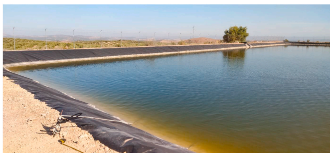
Fig. 3. Example of a typical water irrigation pond existing in Jaén.
