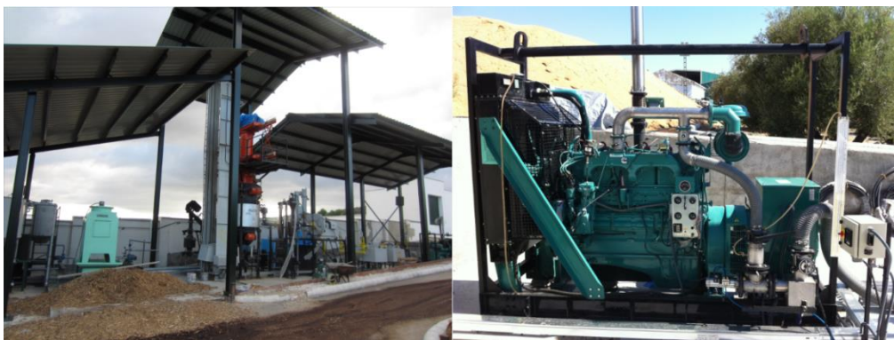
Fig. 18 Gasification plant (left) with a gas motor Cummins ® G855G (right), operated with syngas from the gasification of biomass.
