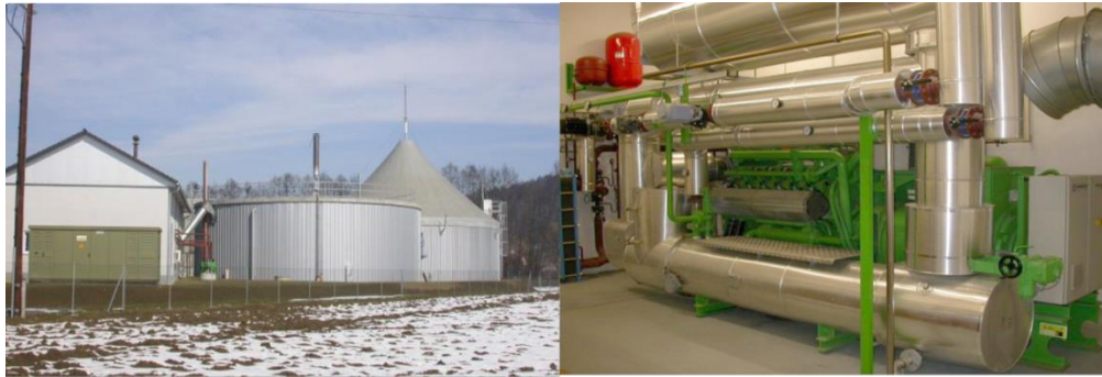
Fig. 19 Biogas plant using anaerobic digestion of manure (left) with a Jenbacher® gas motor (right).
