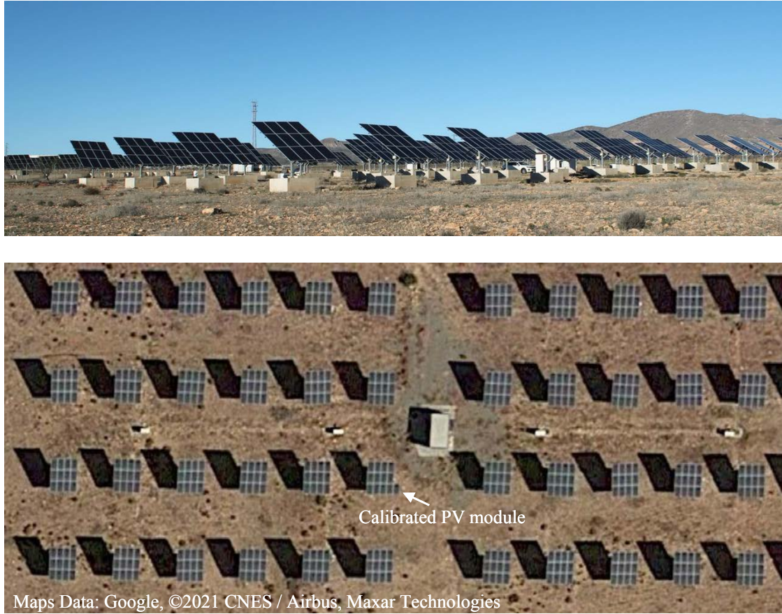
Fig. 3.1. The photovoltaic plant under study in Granada, Spain, has a datasheet nominal power of 109.44 kW. Top: Photo taken at ground level. Bottom: Satellite Image (Latitude: 37.287, Longitude: -3.057).
