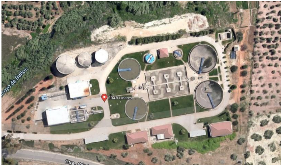
Figure 1 - Wastewater plant in Linares
