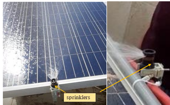
Figure 14 - Water sprinklers used in the project
